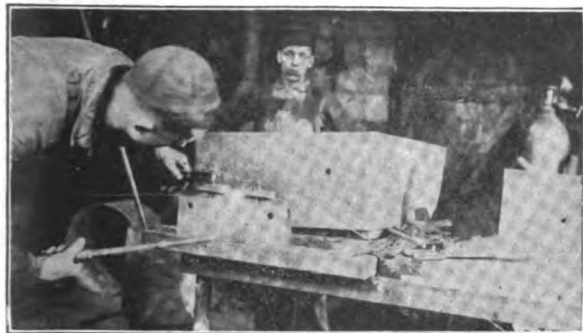
Fig. 2. Heat Both Sides of the Joint Alike
