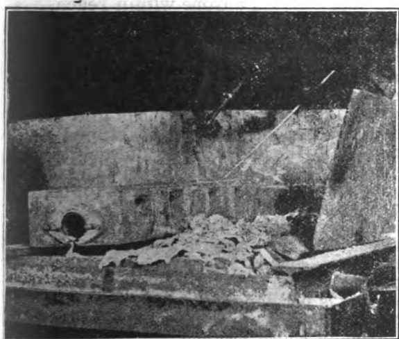
Fig. 1. Preheating a Welding Position.
