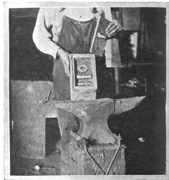
Fig. 3. Details of Hardening Box, with Articles in Place.
