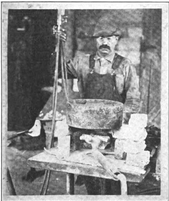
Fig. 3. Arrangement of Preheating Device.
