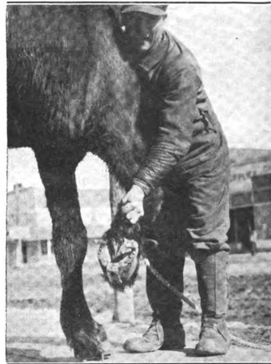
A Photograph Showing the Shoe in Place with the Foot Lifted to Give a Better Idea of the Construction and Application.
