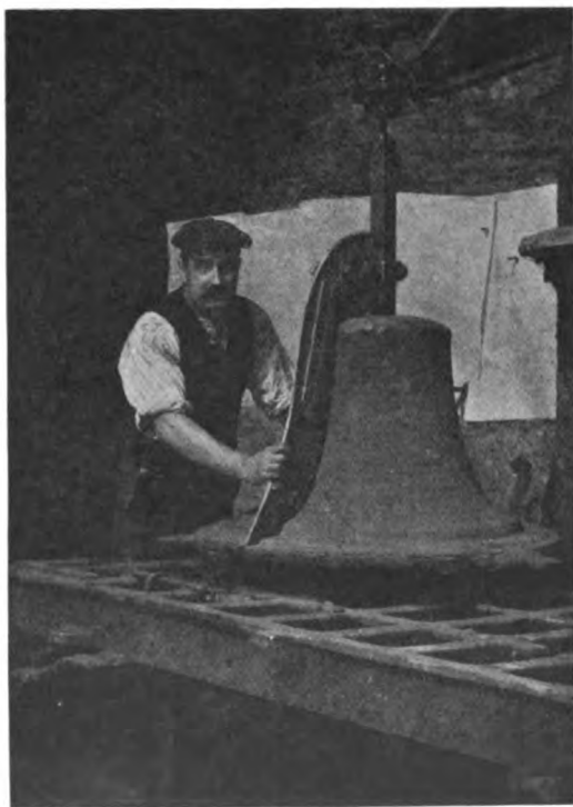
FIG. 199.—Striking up Core for Bell.
